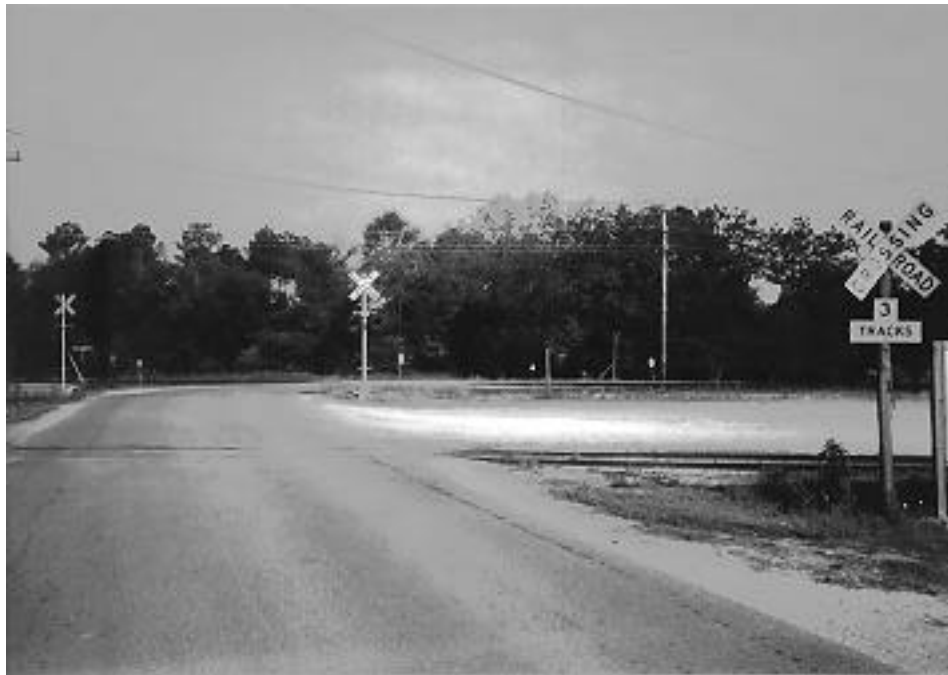
Photo Crosby Road Crossing
